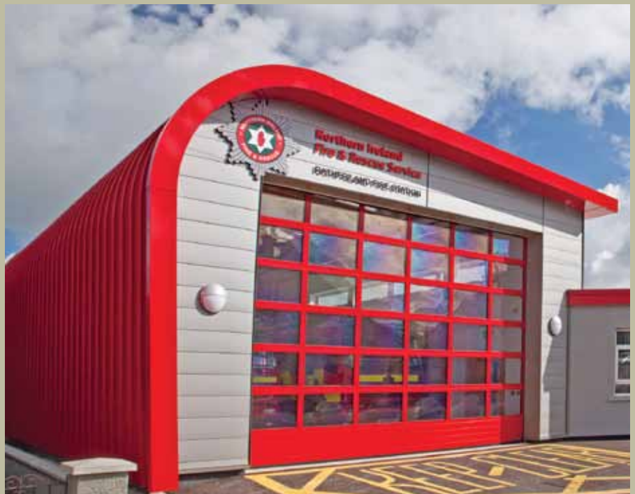
Rathfriland Fire Station, Northern Ireland
